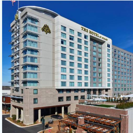
THE HOTEL AT AVALON 9000 AVALON BLVD ALPHARETTA, GA 30009
